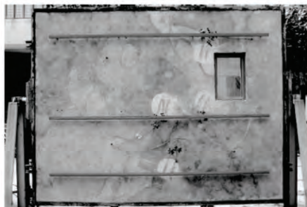
(e) Internal facade of rig wall
